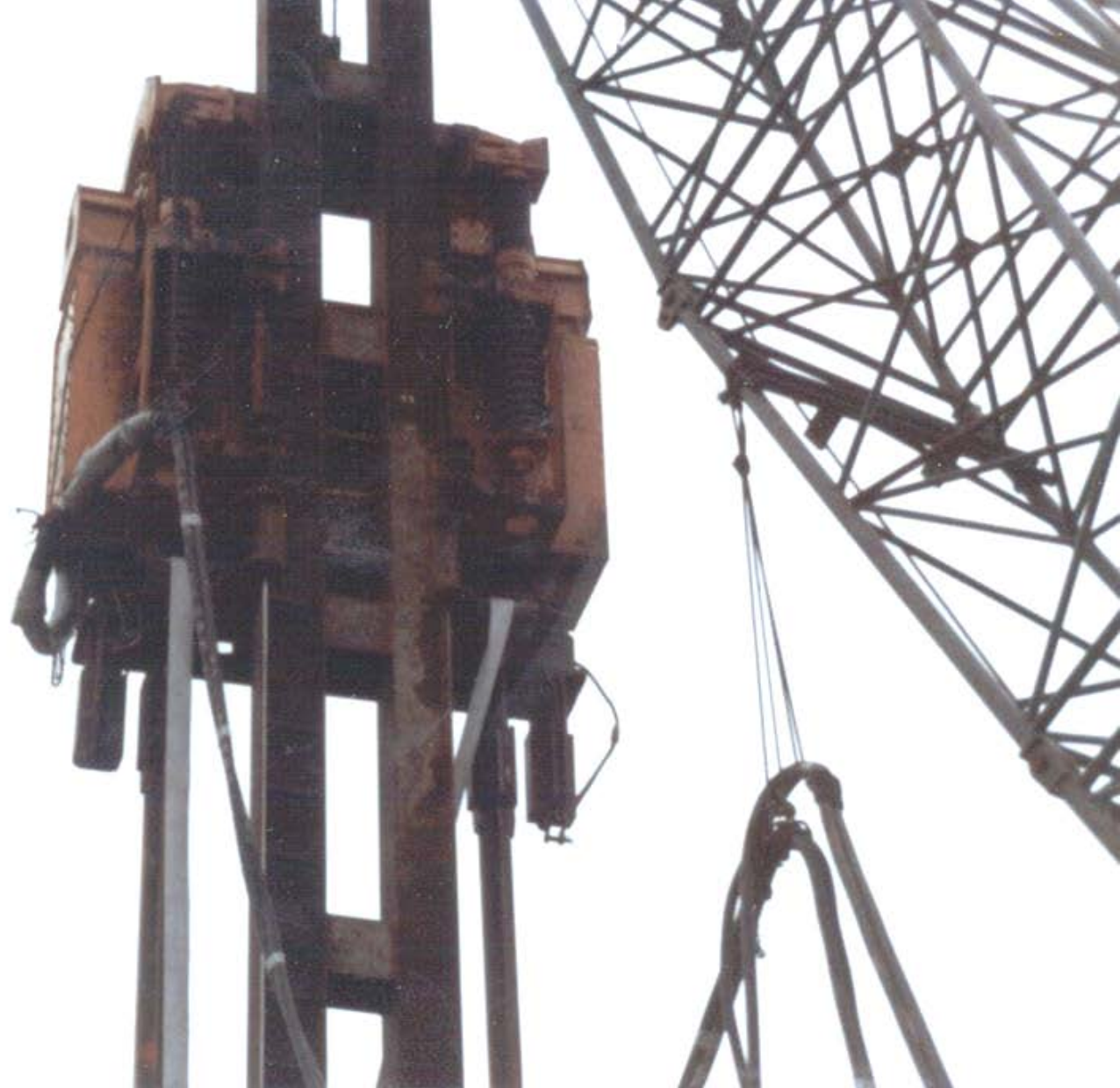
Top drive dual vibro rig driving two wicks at once.
