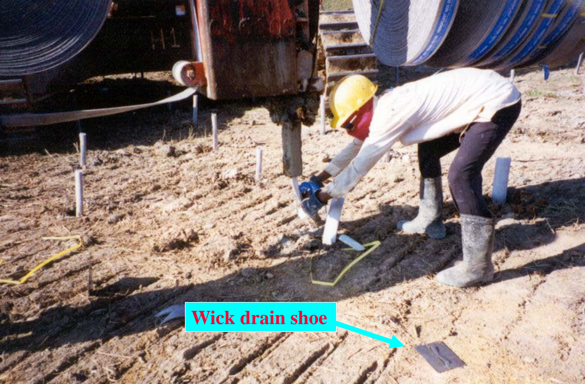
Installing shoes on wick drain
