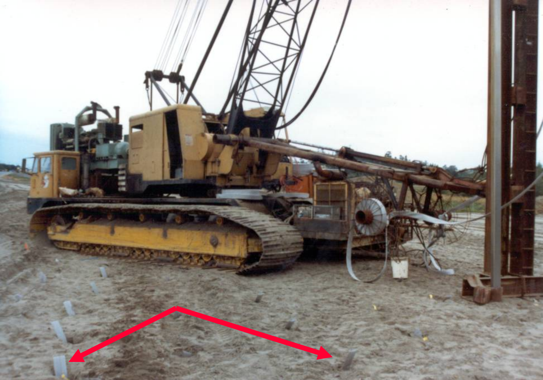
Top drive vibro driving two wicks at once.
