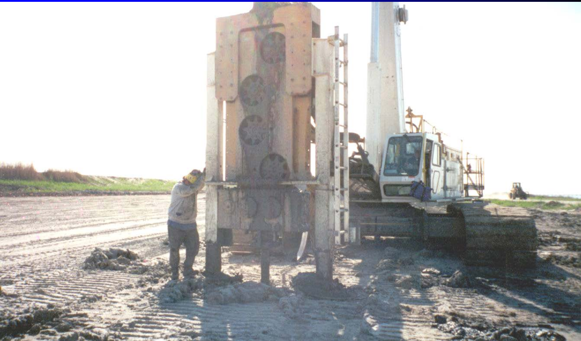
APE bottom drive at Craney Island August 2000
